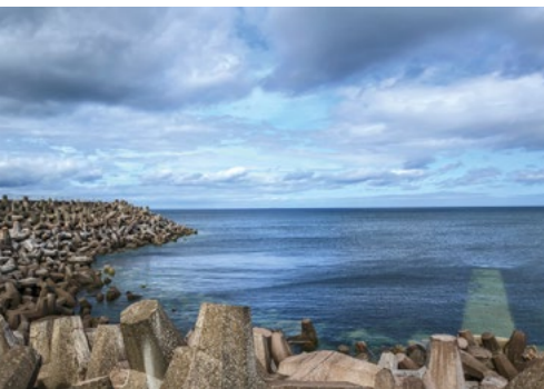
The breakwater at Torness provides an extra line of protection for the station from the North Sea
